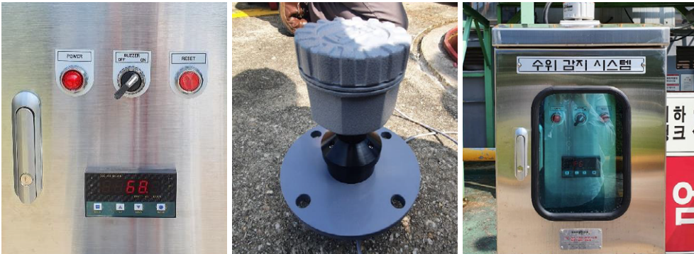
The ultrasonic level gauge and overfill prevention alarm device installed in the toluene storage tank
